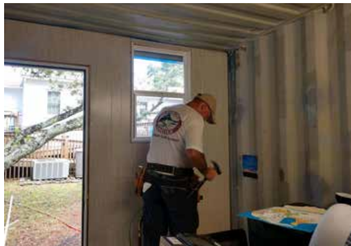
Mike Vercruyse helps finish work on an office.
