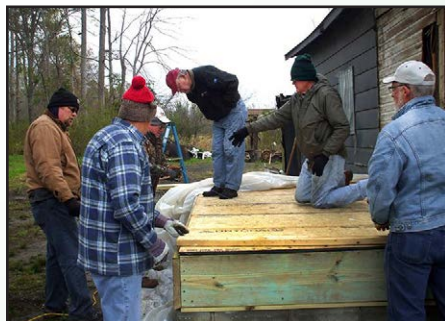
UM Men repair the porch of Allen James.
