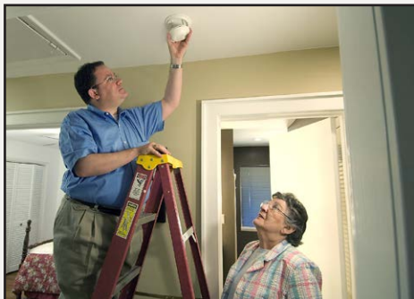
UM Men install free smoke alarms in high risk areas.
